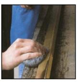
**Distress**Pumice powder and steel wool are used to gently scratch the surface, revealing subtle tones of the red clay.
